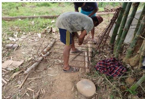
Reinforcement Works by local workers
