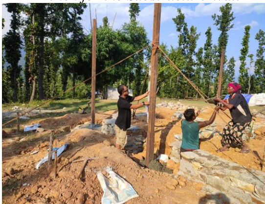
Metal Column Erection
