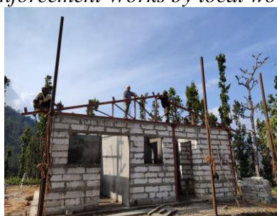
Metal Truss Erection
