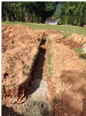
Trench for the Substructure Wall
