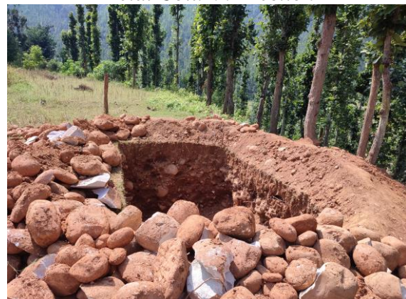
Excavation works for the Septic Tank
