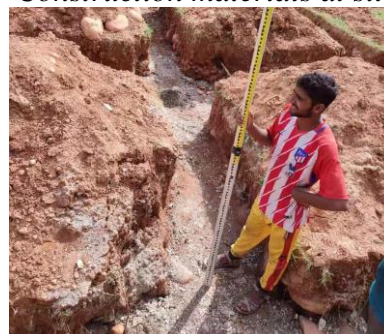
Level checking by technicians
